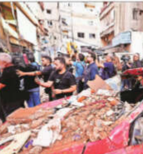
Journalists gather at the scene of a building that was hit by an Israeli airstrike in Beirut's southern suburbs on Tuesday.
